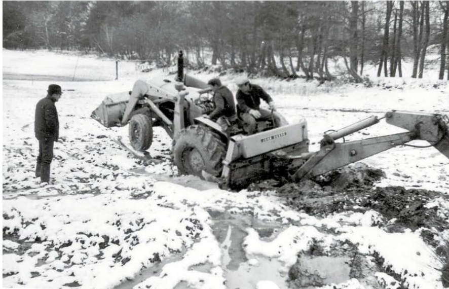
Work begins on reshaping the lake (all rights reserved)
